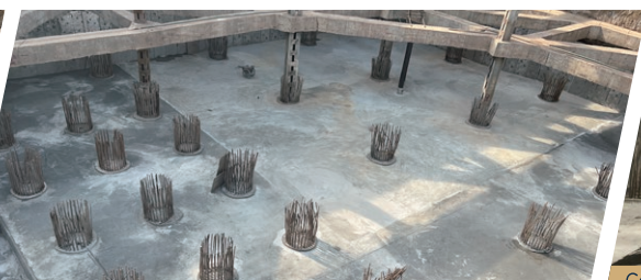
Waterproofing protection work completed 防水保護層已施工完成
