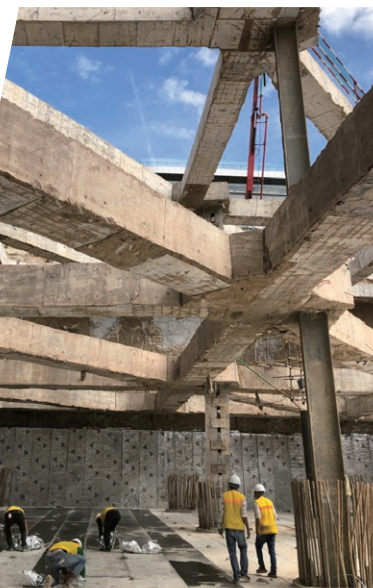
Construction team is working on waterproofing protection work 施工團隊參與防水保護層工作
